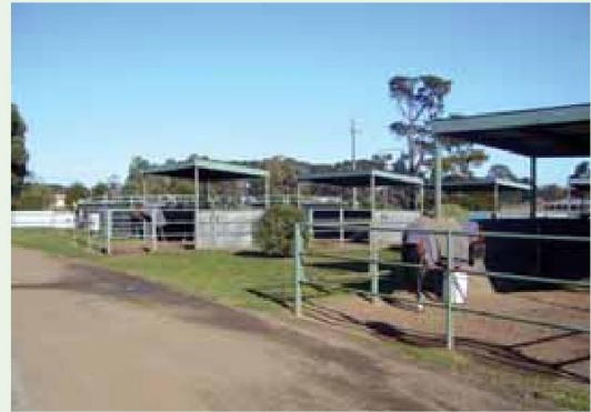
Stable yards are well laid out, tidy and maintained regularly to avoid risk of injuries due to slips, trips and falls.
